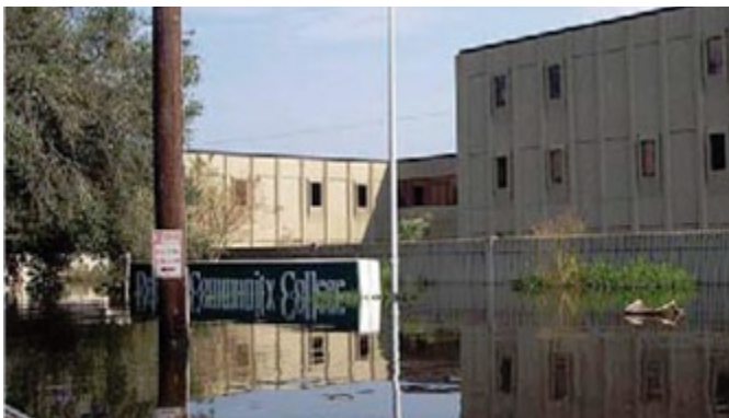
Delgado Community College (immediately after Hurricane Katrina)
